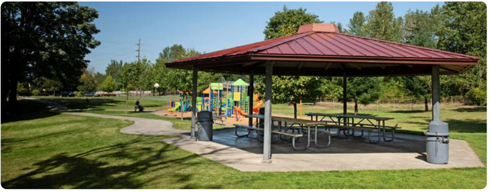
Thomas Teasdale Park Shelter
