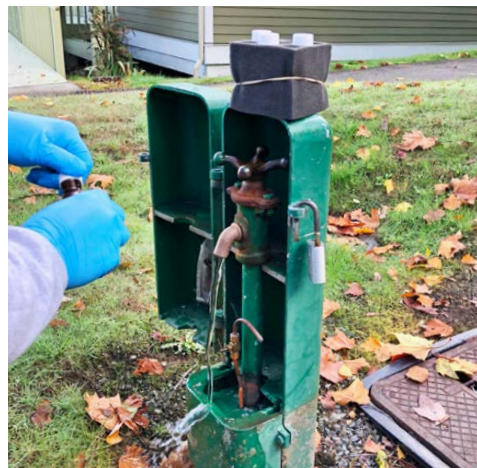
Left: Collecting water samples from a sampling tap located inside the laboratory at the Maplewood Treatment Plant. Right: Renton Water Treatment Operator collecting water samples at a dedicated sampling station.
