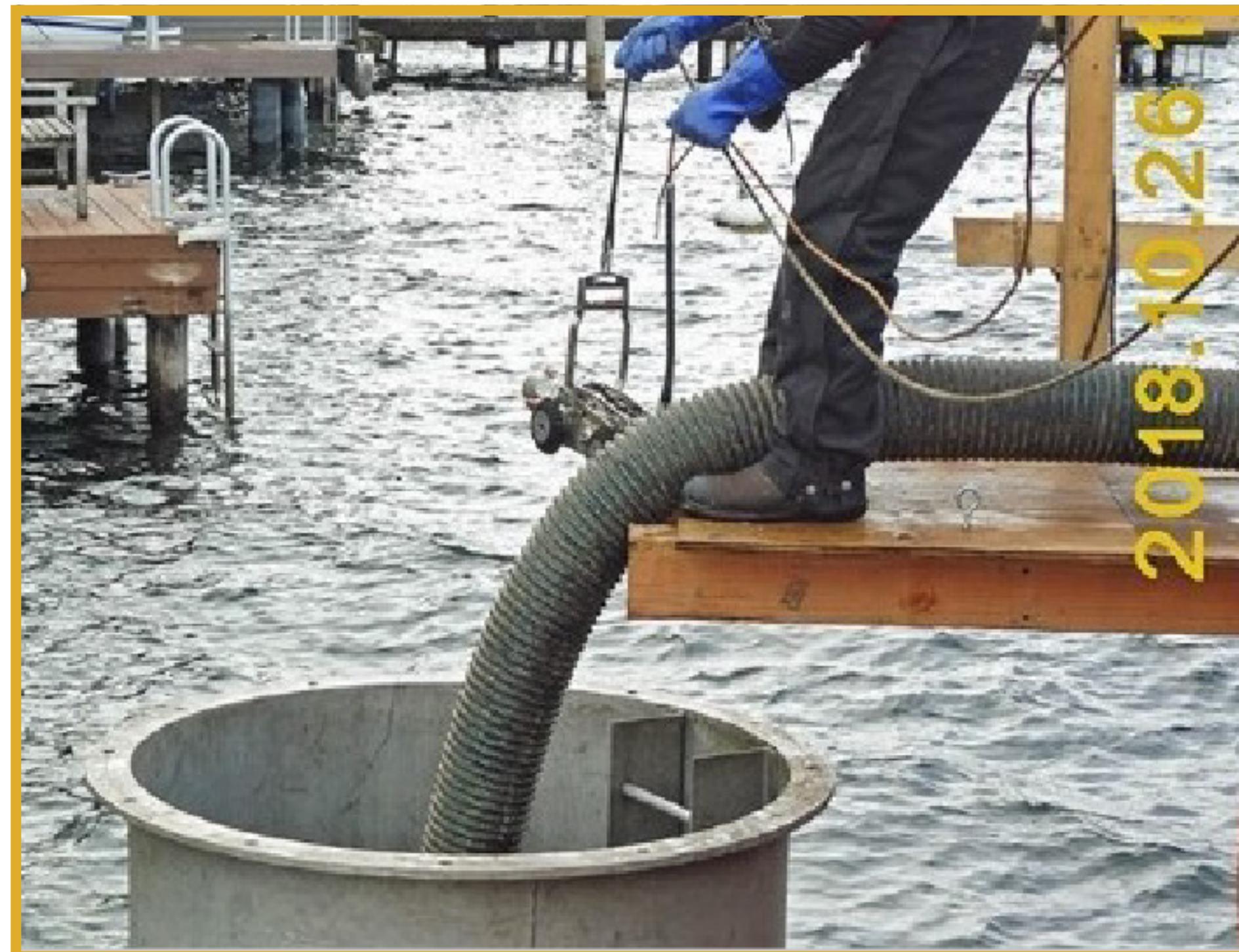
Lakeline cleaning and inspection.
