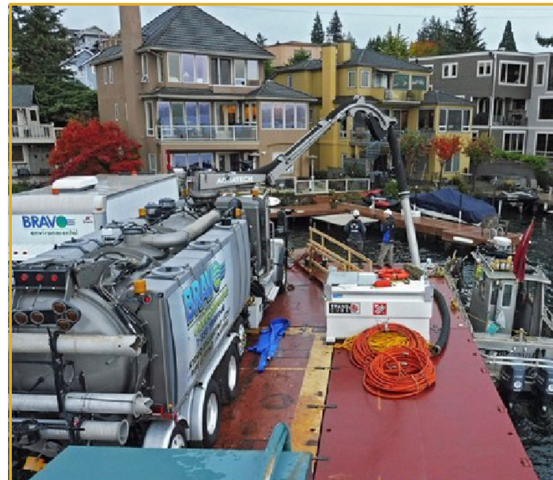
Barge and equipment used for Lakeline cleaning/inspections.
