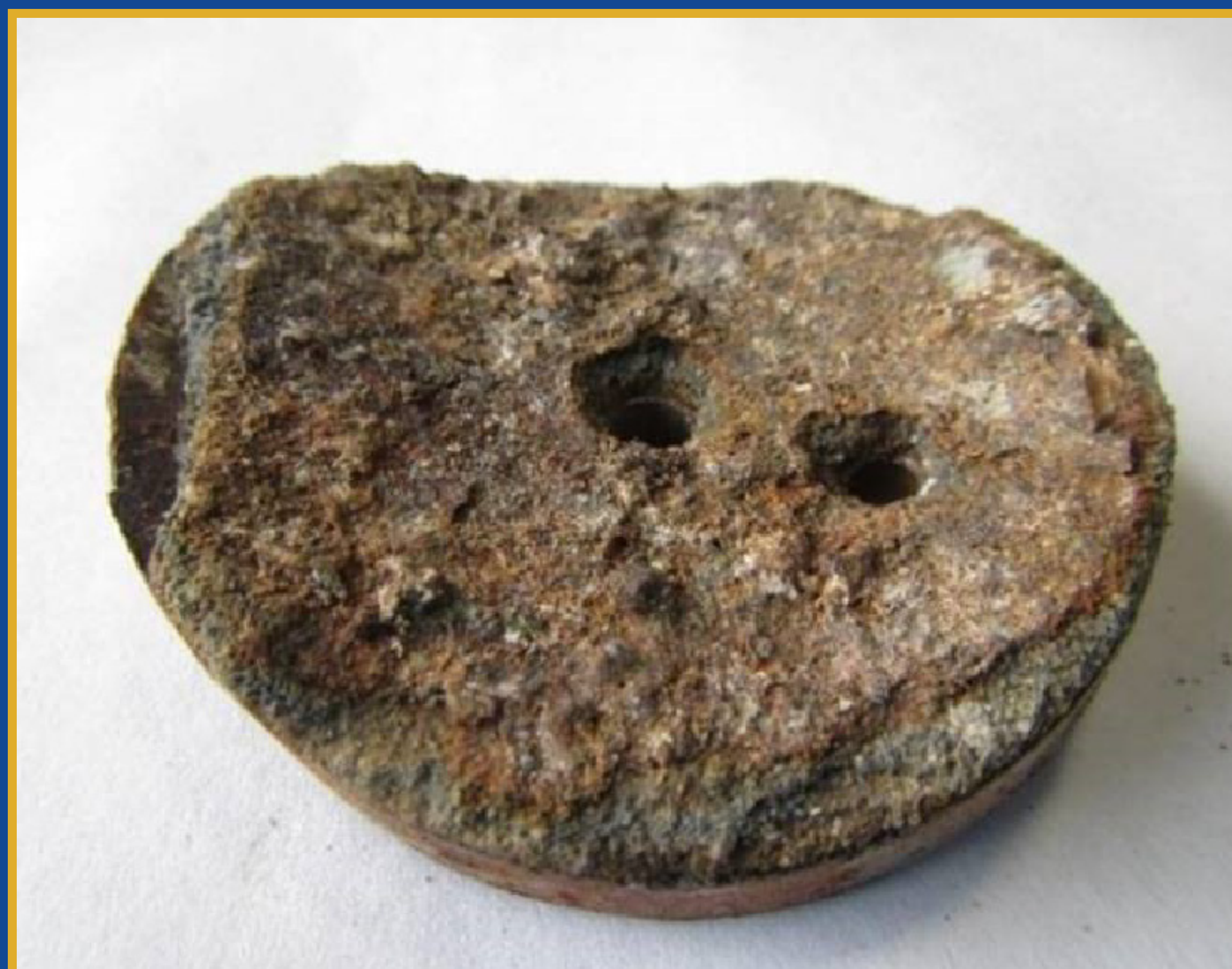
Corroded piece of the Lakeline pipe.
