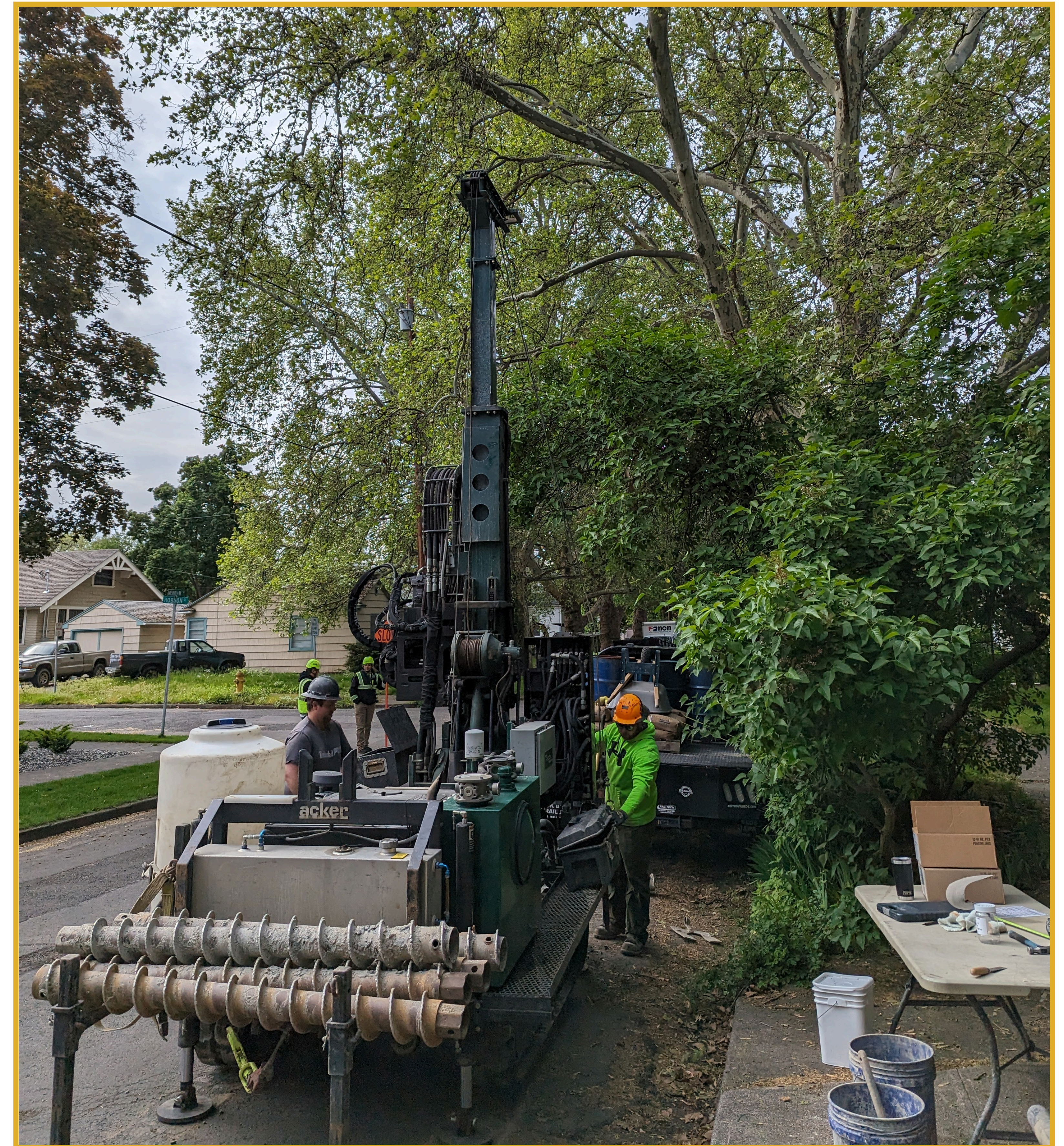
Drill rig used to obtain soil borings.
