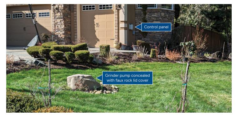
Example of a grinder pump station and control panel at a home located in Soos Creek. These homeowners opted for a decorative rock to conceal the lid. The control panel is located on the side of the garage.
