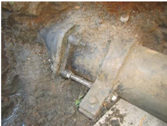
Photo C-7. 4"x8" reducer with mechanical joint
