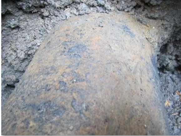
Photo C-3. Close up of top of Lakeline
