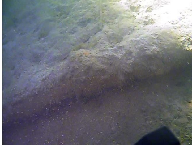
Figure 6.1-10 Unsupported Bottom of Lake Line where Shoreline has Steep Drop-Offs
