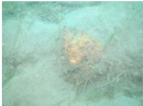
Photo C-55. Corrosion scale/tuberculation underneath dirt/debris
