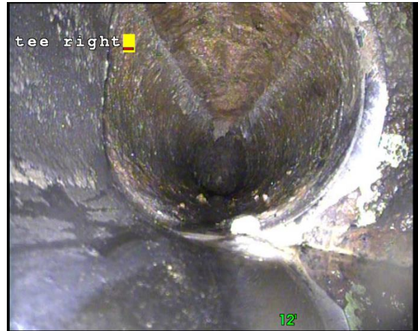
Photo 2-23. Apparent air pocket in lateral
