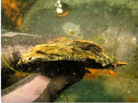
Photo C-62. Scale/tuberculation removed from pipe surface
