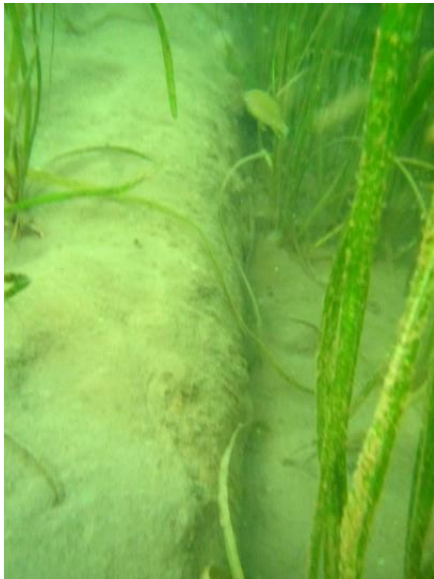
Photo C-68. Mainline covered in dirt/debris; surrounded by vegetation
