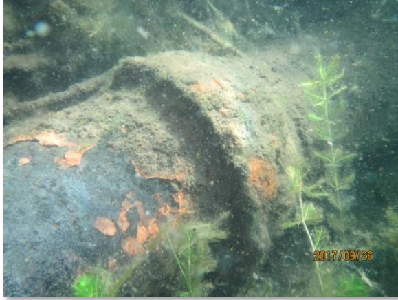
Photo C-23. Bell/spigot joint on north end of exposed reach
