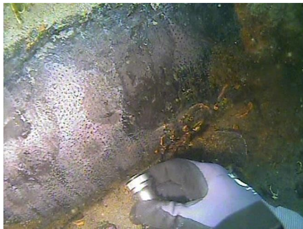
Figure 6.1-6 Typical Pipe Surface
