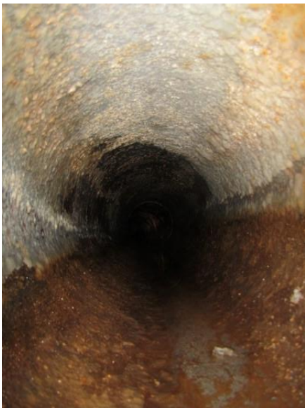
Photo C-13. Interior of Lakeline looking downstream
