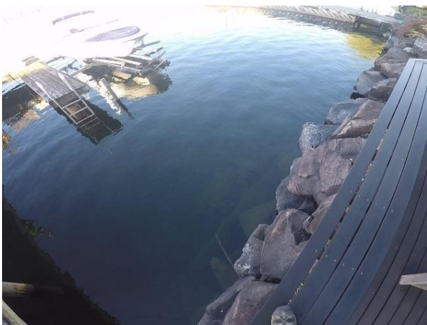
Figure 6.1-9 Rip-Rap Directly Adjacent to and Above Lake Line at 2811 Mountain View Avenue North
