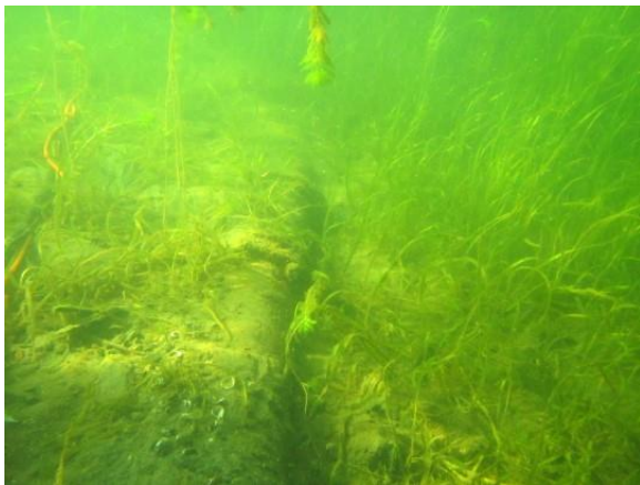
Photo C-54. Offshore side of mainline exposed
