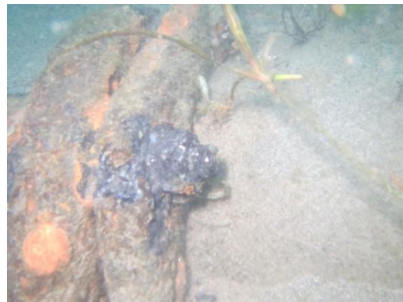
Photo C-48. Nuts, bolts glands of mechanical joints with corrosion but in fair condition
