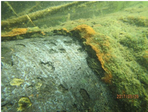
Photo 2-3. Surface of mainline after scaling and corrosion was removed
