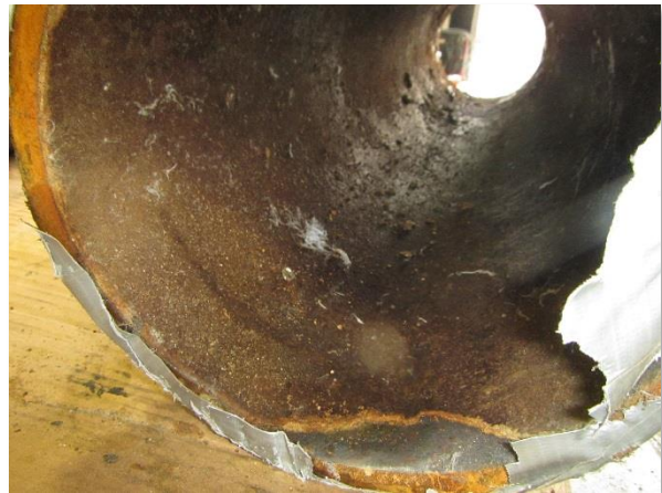
Photo 3-4. Cement mortar lining on interior of Manhole 5 sample.
