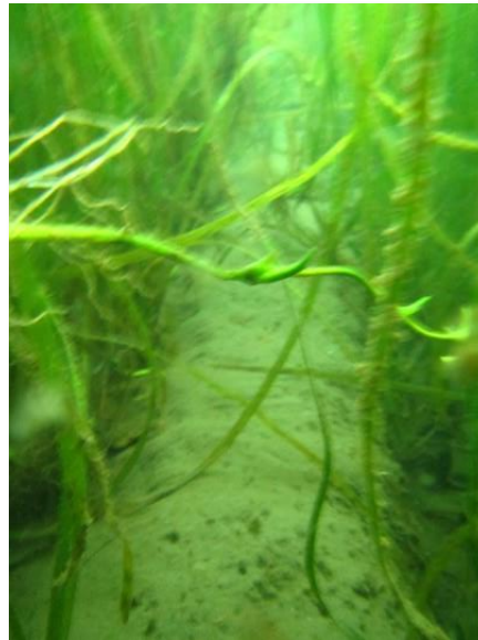
Photo C-69. Mainline covered in dirt/debris; surrounded by vegetation
