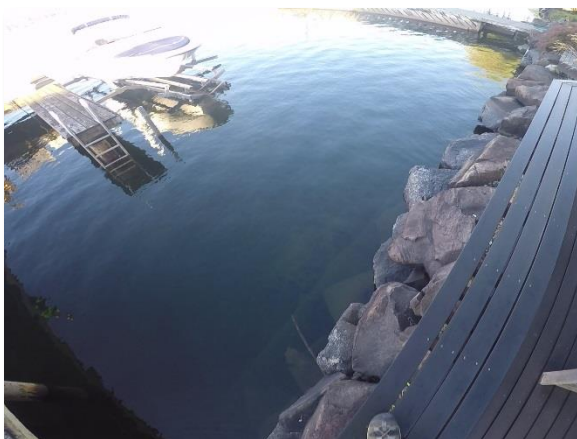
Photo 2-9. Rip-rap directly adjacent to and above Lakeline at 2811 Mountain View Ave. North
