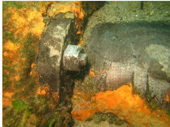
Photo 2-8. Typical mechanical joints at wye and tee fittings for lateral connections
