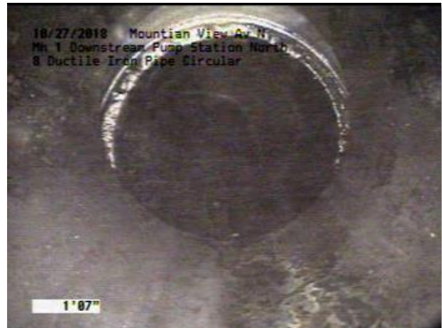
Photo 3-18. Typical offset joint.
