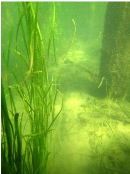
Photo C-72. Mainline sits only inches from dock pilings
