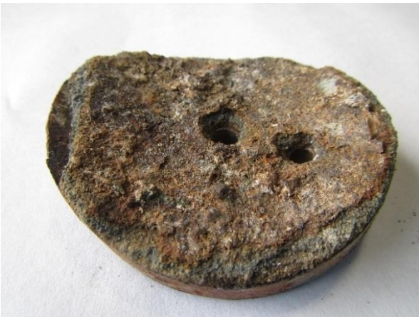
Figure 6.3-7 Deteriorated Cement Mortar Lining on Lateral Coupon
