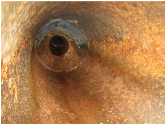
Photo C-11. Interior of Lakeline looking towards reducer
