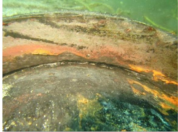
Photo C-63. Side view of bell portion of push-on joint
