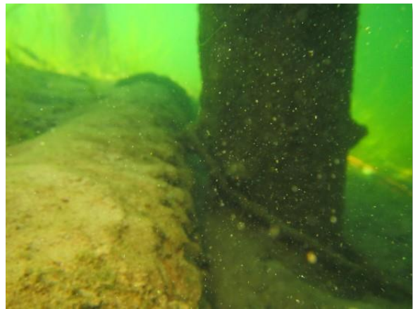
Photo C-67. Pipe sits only a few inches from dock pilings
