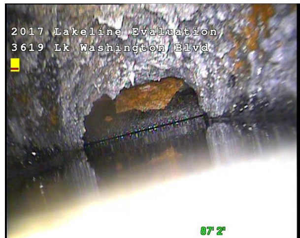
Photo 2-13. Wye or tee fitting connection to mainline at 3619 Lake Washington Blvd. North
