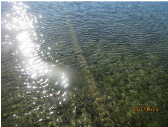
Photo C-25. Mainline exposed in shallow water (less than 3 feet deep)
