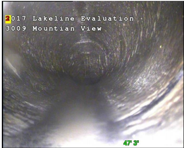
Photo 2-22. Typical lateral interior
