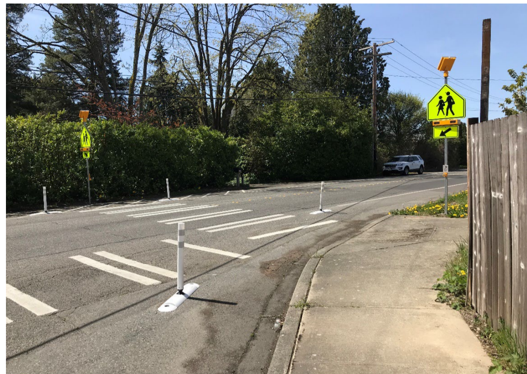
*Picture: Benson Rd S/S 29th St where crossing improvements, including installation of a Rectangular Rapid Flashing Beacon (RRFB), have been completed.
