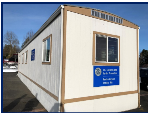
11. Exterior of USCBP Trailer
