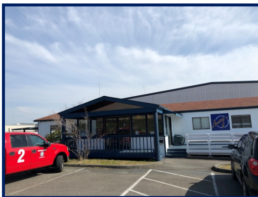
17. BEFA office exterior
