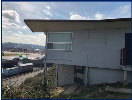
1. Exterior of 300 Rainier Avenue
