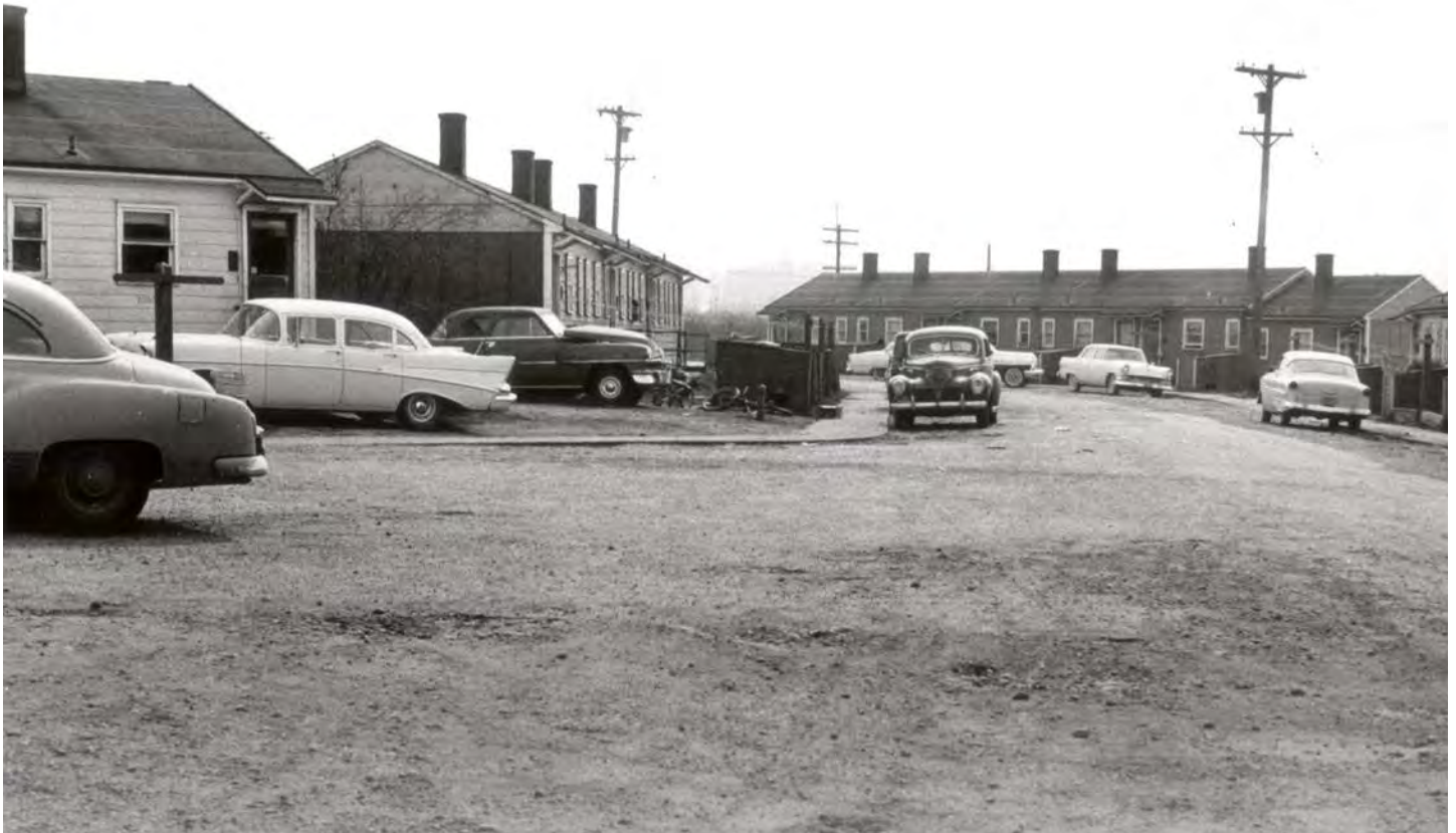
Fourplexes in the Renton Highlands, 1958. Four families shared one building; the neighbors all used a common yard. (RHM# 1998.046.9790)
