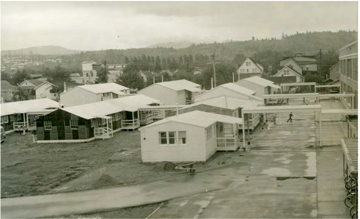
Portable classrooms behind Renton High School, 1945. To accommodate all the extra students, the school district purchased six U.S. Army barracks to repurpose as classrooms. (RHM# 1980.096.1409)
