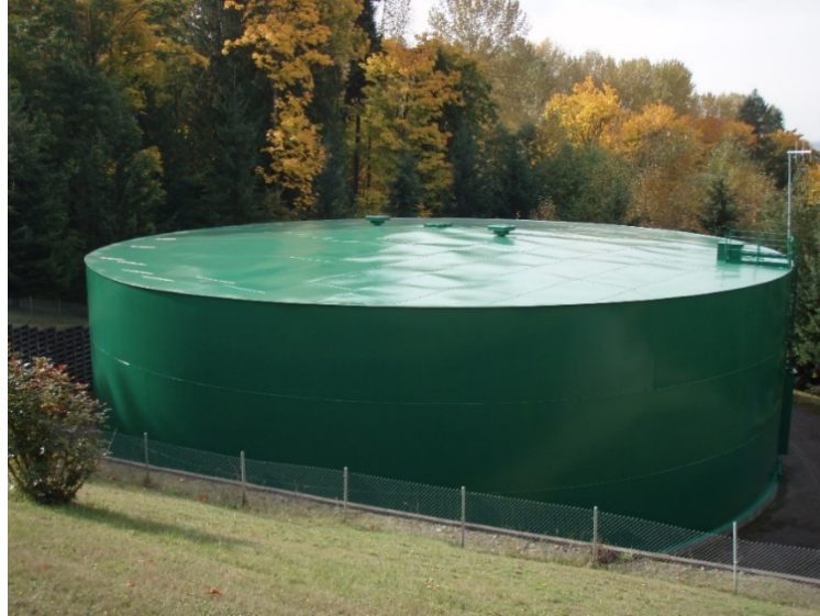
South Talbot Reservoir – 1.5 MG
