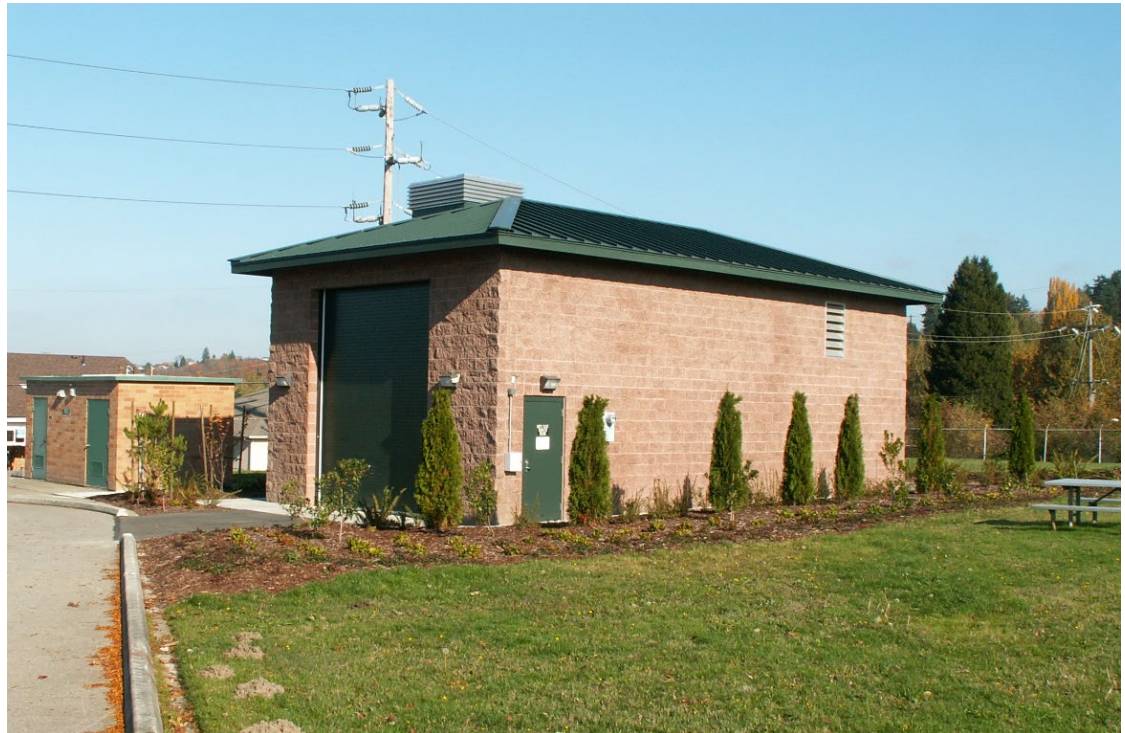
North Talbot Booster Pump Station
