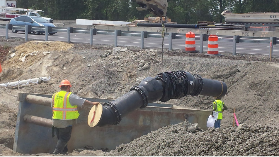
Pipeline -Flex Joint Installation
