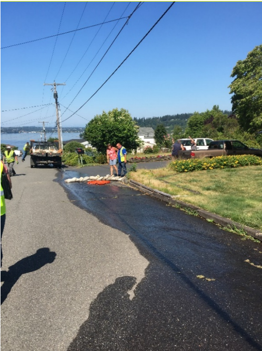
Flow Management during fire flow tests
