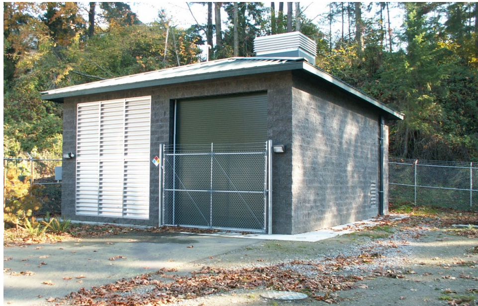
Mt. Olivet Booster Pump Station
