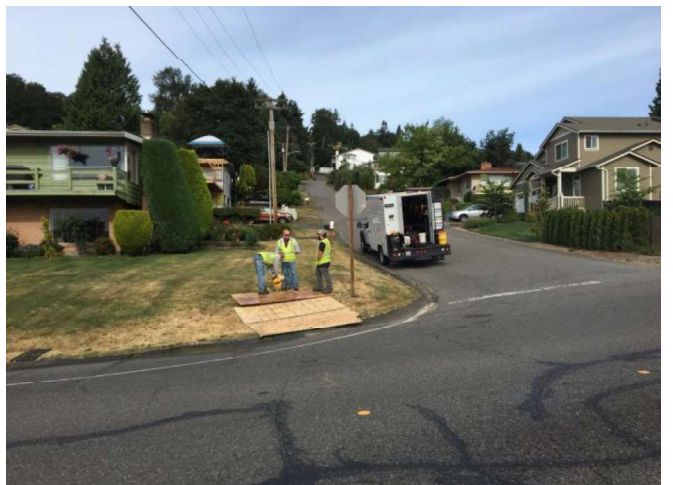
Diffuser setup of flowing hydrant F1
