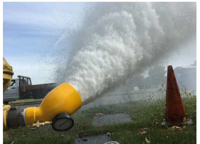
Diffuser setup and flowing the hydrant F1
