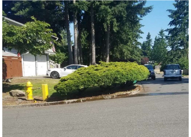
Logger setup for pressure hydrant 1
