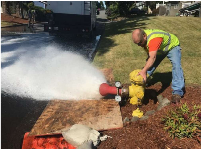
Diffuser set up and flowing on flow hydrant F1
