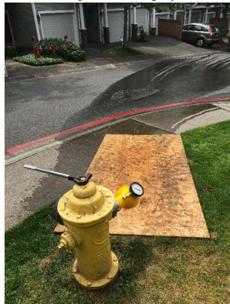
Diffuser setup of flowing hydrant F1
