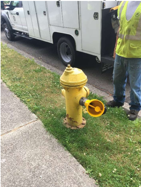
Diffuser setup of flowing hydrant F1
