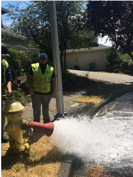
Diffuser setup of flowing hydrant F1
