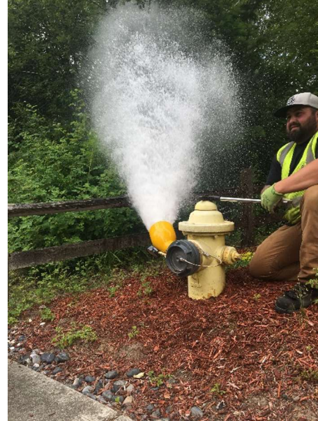
Diffuser setup of flowing hydrant F1
