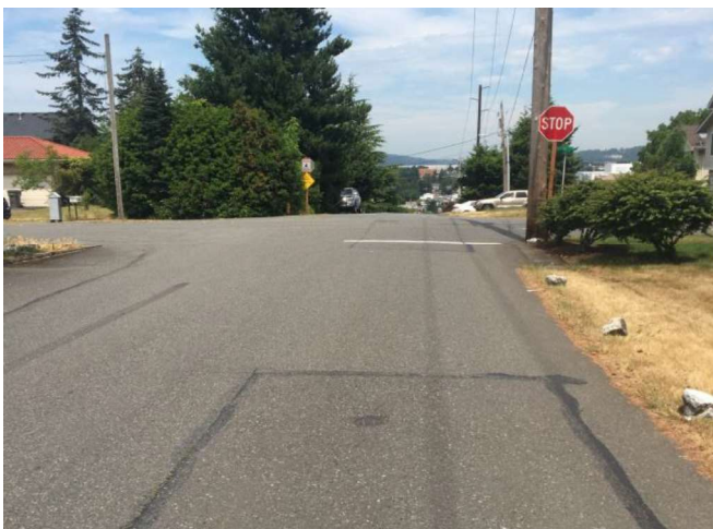
Area surrounding flowing hydrant F1
