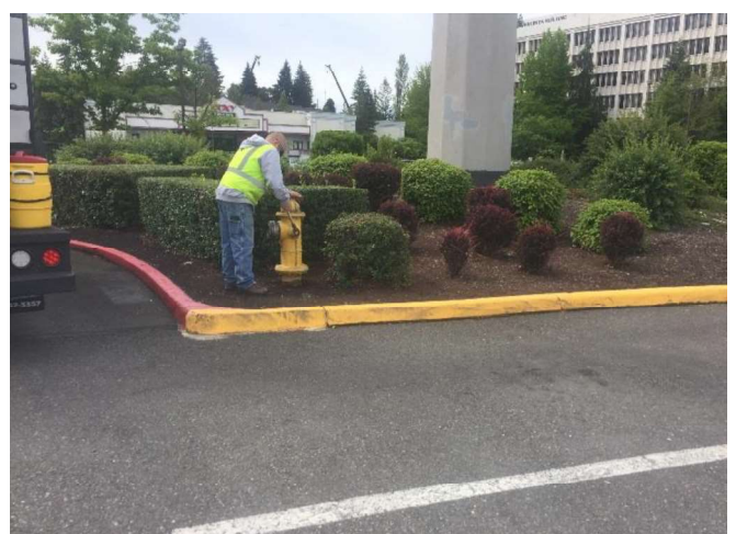
Diffuser setup of flowing hydrant 2 (F2)
