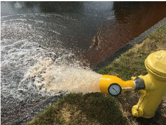
Diffuser setup of flowing hydrant F1
