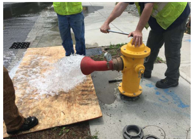
Diffuser setup of flowing hydrant F1
