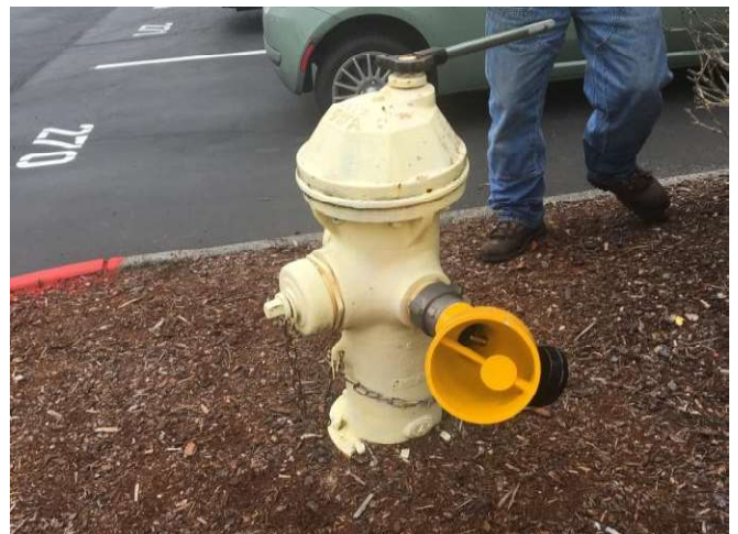
Diffuser setup of flowing hydrant F1
