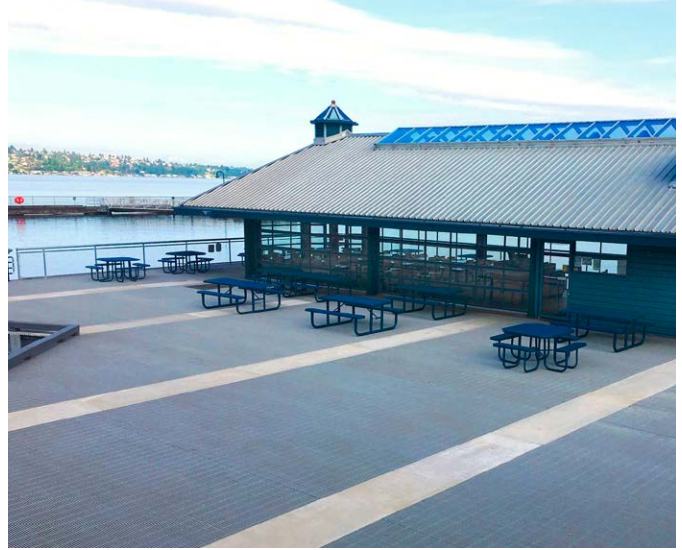
After: Structural repairs and light-penetrating decking
