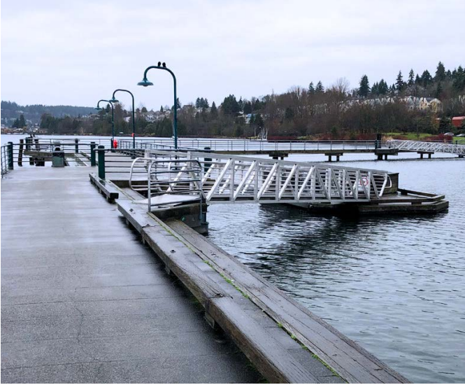
Before: Concrete decking to be replaced and picnic floats retrofitted
