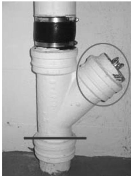
*Main sewer cleanout in a house with a basement. The top of the test plug should be below the blue line*
